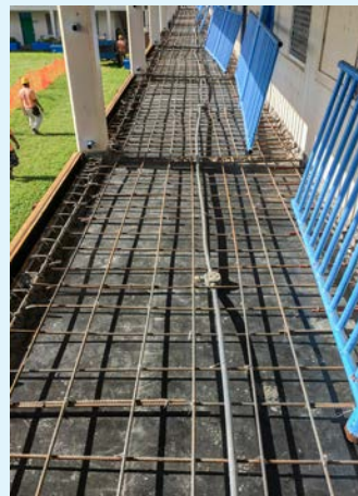
Above, left: Rusted railings are being replaced. Second from left: Existing concrete has cracks and spalling. Third from left: New rebar is laid to support new concrete flooring. Top, right: A crew from E&W Construction pours new concrete.
