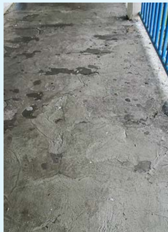
Above, left: Rusted railings are being replaced. Second from left: Existing concrete has cracks and spalling. Third from left: New rebar is laid to support new concrete flooring. Top, right: A crew from E&W Construction pours new concrete.
