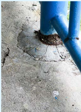
Above, left: Rusted railings are being replaced. Second from left: Existing concrete has cracks and spalling. Third from left: New rebar is laid to support new concrete flooring. Top, right: A crew from E&W Construction pours new concrete.
