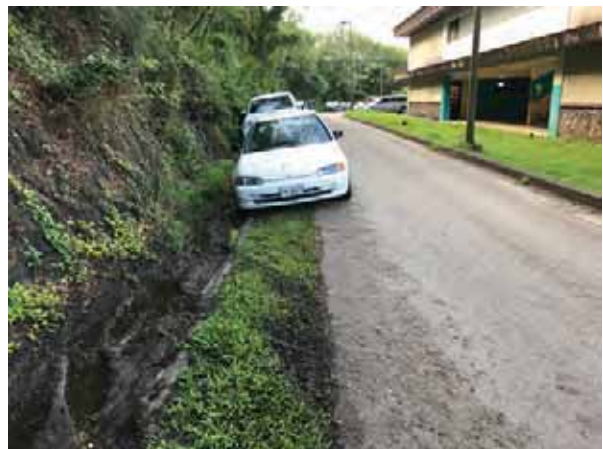
Figure 26: Vehicles parked within a drainage structure damages the planned function of the swale and causes storm water to backup and flood to other areas of campus. These parked cars are also blocking the fire access lane.
