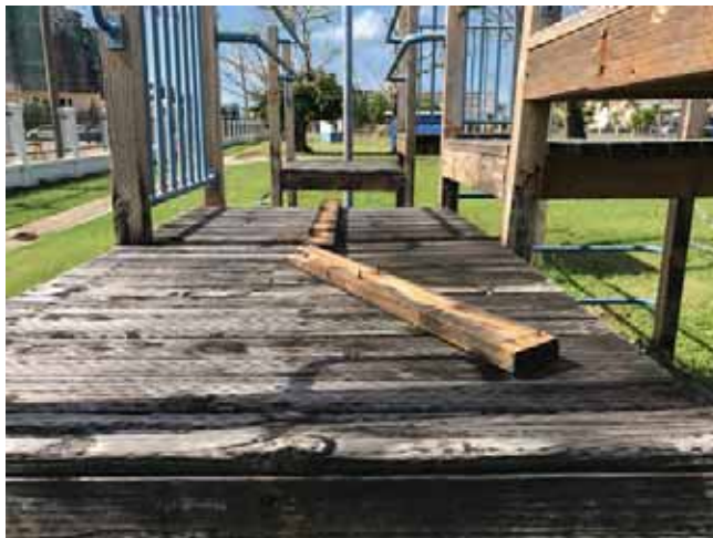
Figure 41: Play structure is compromised by extensive wood rot. Exposed nails are a safety hazard and should be removed immediately. Grass is not a safe surfacing for fall protection; a certified resilient play surface is recommended.
