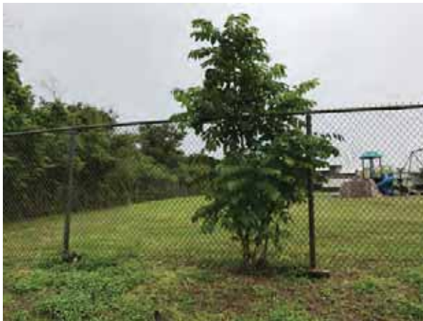
Figure 23: Young tree growing along the fence line will eventually damage the fence unless it is removed soon.
