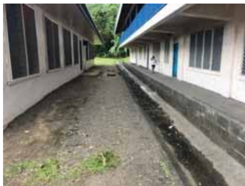
(Left Photo) Re-construct flat concrete swale to flow freely towards the grass swale beyond.
