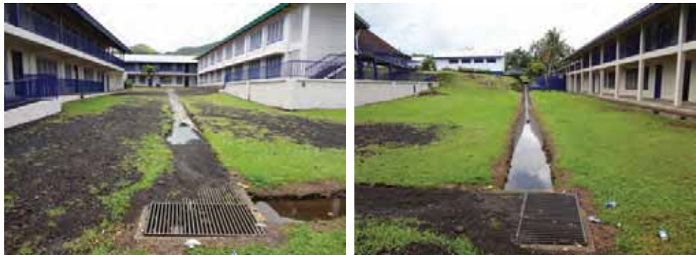
Figure 9: Trench drains are easily clogged with dirt and vegetation. Periodic inspection and cleaning is needed to prevent flooding.
