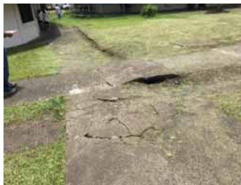
(Left Photo) Re-construct flat concrete swale to flow freely towards the grass swale beyond.
