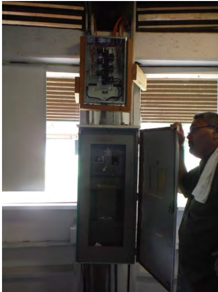
Building 10 – New panel improperly installed, height exceeds Code acceptable mounting height
