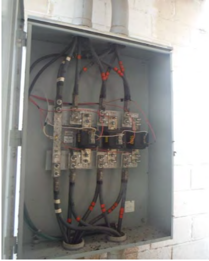
Building 09 – Electrical equipment cabinet is not secured exposing live electrical bussing
