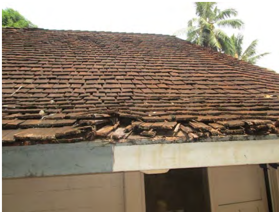
Deteriorated wood shakes
