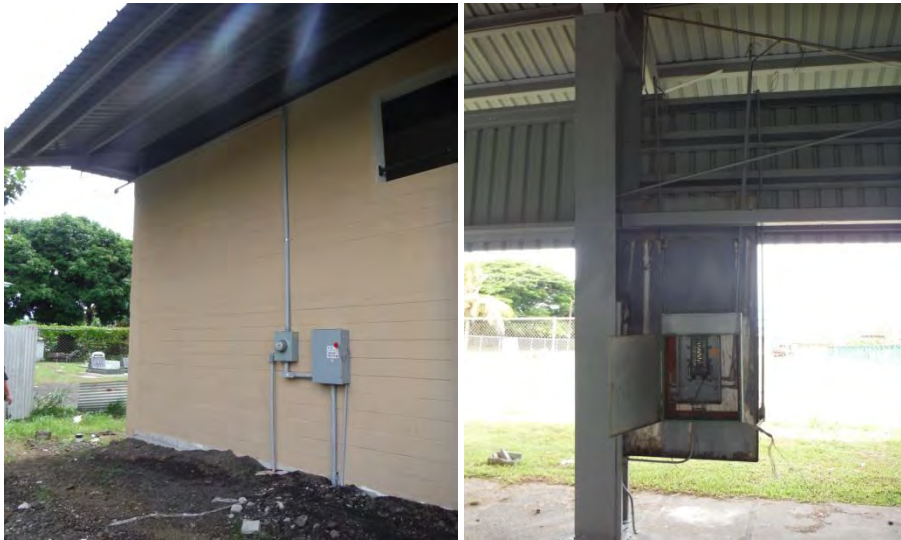
Building 10 – New panel improperly installed, height exceeds Code acceptable mounting height
