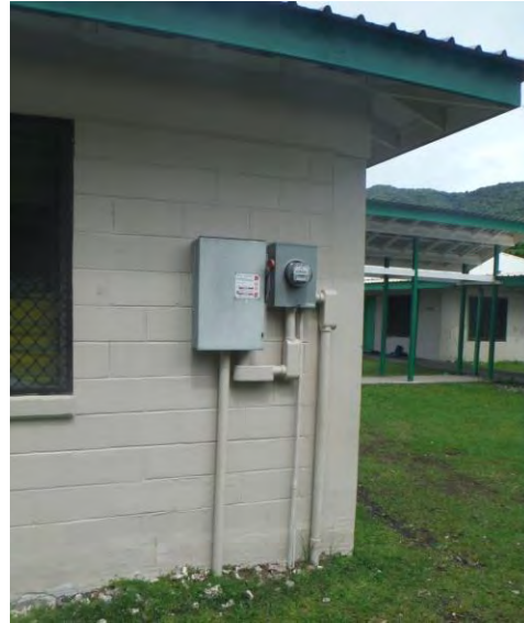
Building 03 – New ASPA Electrical Service/Meter
