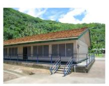
Figure 2-15 – Lauli'i Elementary. Masonry wall building with wood framed roof.
