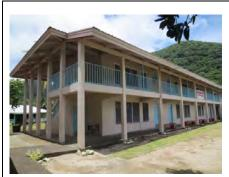
Figure 2-14 – Masefau Elementary. Concrete frames with concrete infill walls and wood roof decking.
