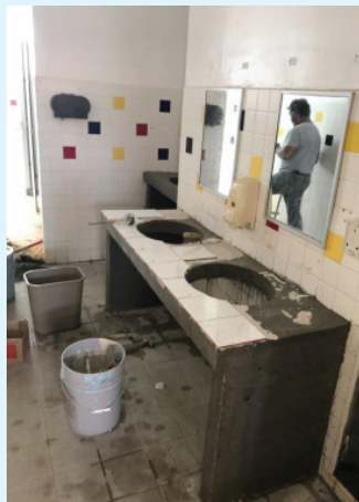
Above, left: Wood countertops are being replaced with more durable materials (steel-reinforced, cast-in-place concrete). Above, right: Concrete lavatories with tile finish.
