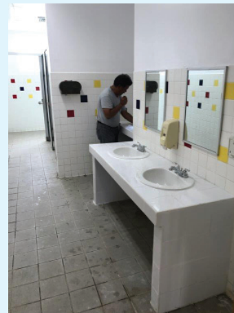
Above, left: Wood countertops are being replaced with more durable materials (steel-reinforced, cast-in-place concrete). Above, right: Concrete lavatories with tile finish.
