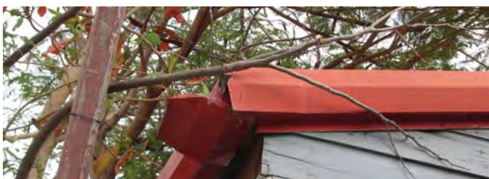
Iguanas and other pests enter classroom attics through holes created by damaged flashing.
