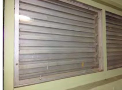
Plexiglass covering windows help retain cooled air but also eliminate the possibility of natural ventilation.
