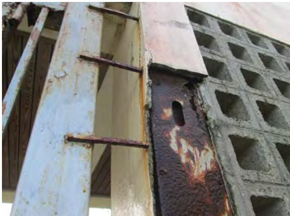
Corrosion of steel column by marine environment.
