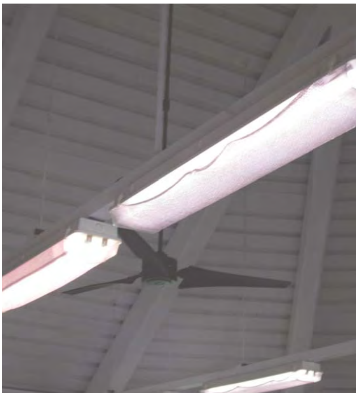
Above: Users wrap fabric around lighting because the room feels too bright and hot. Instead, differential light controls would allow users to turn off or dim a portion of the lights.
