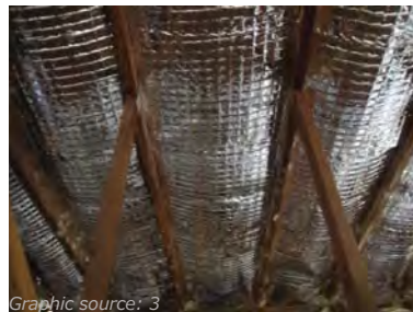
Radiant barrier insulation draped between trusses
