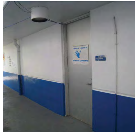
Unpainted aluminum door resists corrosion well.
