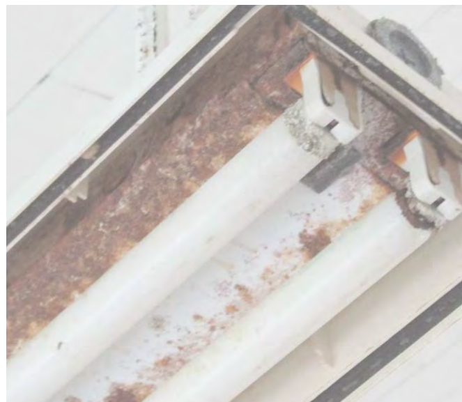
Corroded light fixture; missing light cover.
