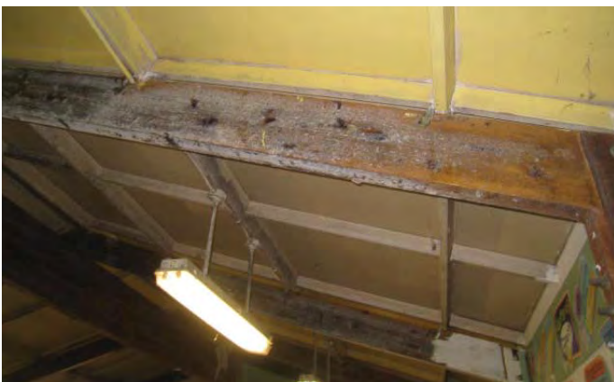
Mold on exposed roof framing
