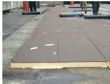
Foam board insulation on roof
