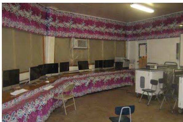
Photos: Classrooms have different reasons for blocking windows. Left: Windows blocked to reduce glare and reduce air-conditioned air leakage. Right: Windows blocked to reduce glare but also blocks natural ventilation. Far Right: As a temporary solution, clear plastic is used to reduce air-conditioned air leakage while allowing flexibility for natural daylighting.
