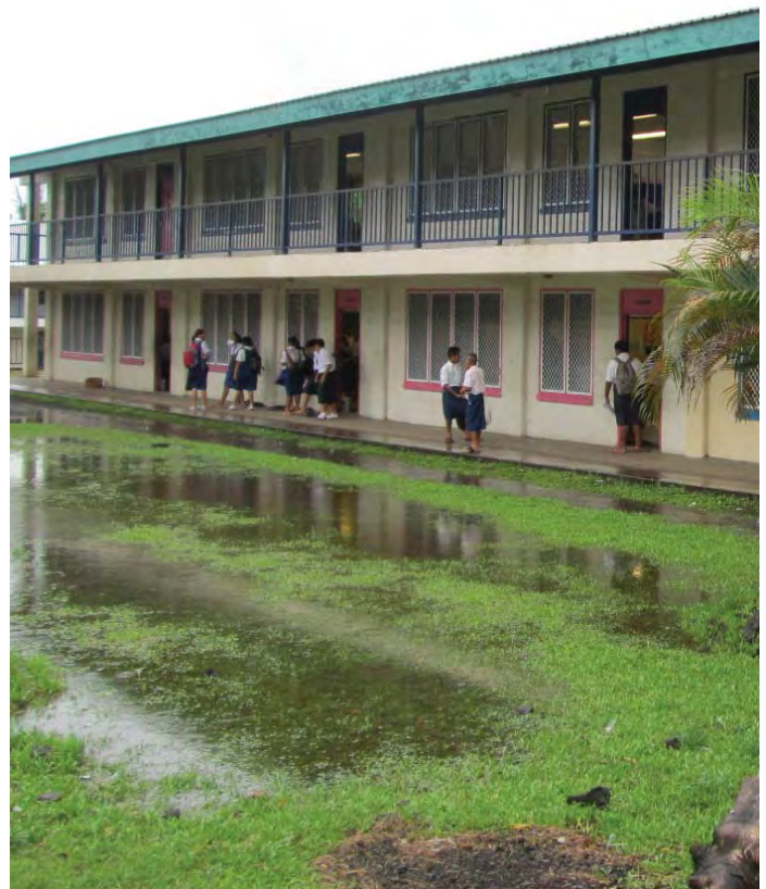
Poor site drainage stimulates mold growth within classrooms
