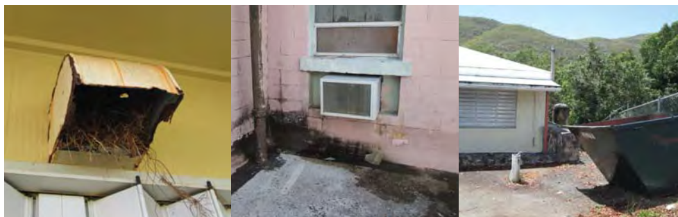
Left: Bird nest and debris in air vent. Middle: Mold growing near window AC. Right: Trash area next to a classroom window
