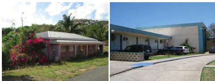
Left: Overgrown landscaping can damage structure, trap moisture, and allow pests to enter. Right: Parking too close to classroom windows and AC.
