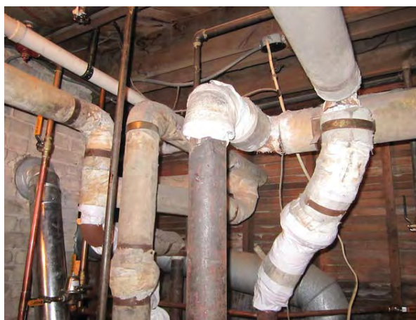
Asbestos is found in many building products, including pipe insulation.
