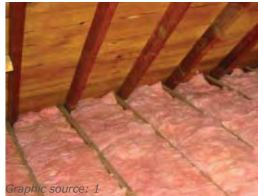
Batt insulation in attic
