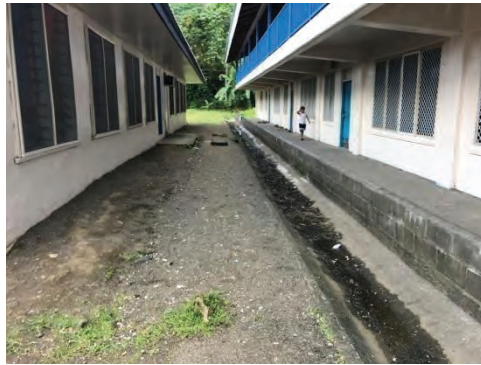
(Left Photo) Re-construct flat concrete swale to flow freely towards the grass swale beyond.
