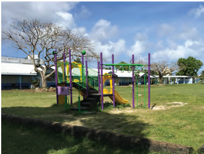
Figure 40: Sand or grass is not a safe surfacing for fall protection; a certified resilient play surface is recommended.
