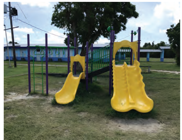
Figure 40: Sand or grass is not a safe surfacing for fall protection; a certified resilient play surface is recommended.
