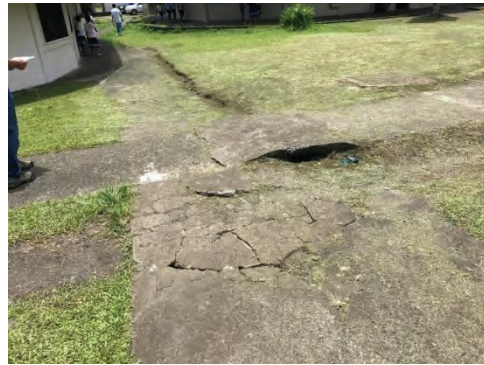
(Left Photo) Re-construct flat concrete swale to flow freely towards the grass swale beyond.
