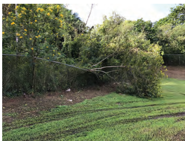
Figure 22: Fallen trees and overgrown vegetation has damaged section on perimeter chainlink fencing.
