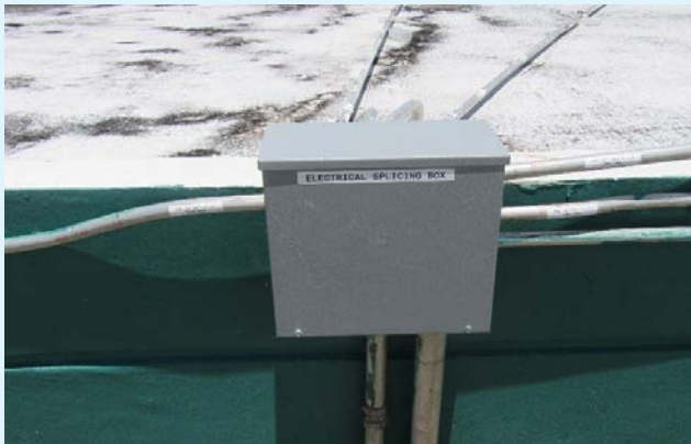
New NEMA-type electrical pull box installed by local contractor Kinden Corporation
