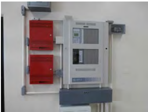
Fire alarm panels at Building 11, Gymnasium
