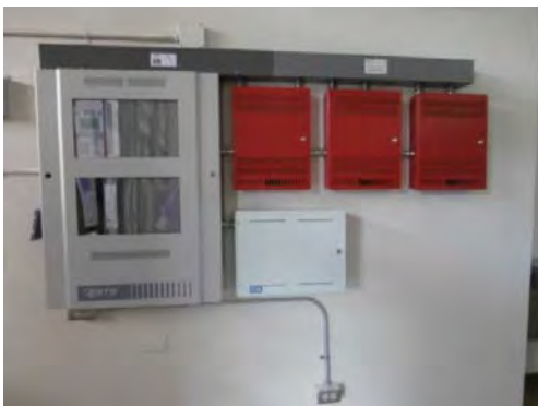
Fire alarm panels at Building 12, Auditorium
