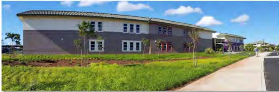
Precast concrete structure, wall panels and double tees
