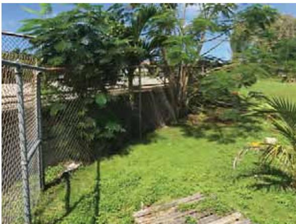
*Figure 24: Trees growing along the fence also disrupt the drainage swale and should be removed.*
