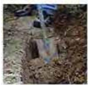
Dig holes and trench for pipe and catch basins. Dry fit (no glue) the entire drainage system from the catch basin to the pop-up emitter. Measure and cut all pipe to necessary lengths. After completing each step, glue parts together.
