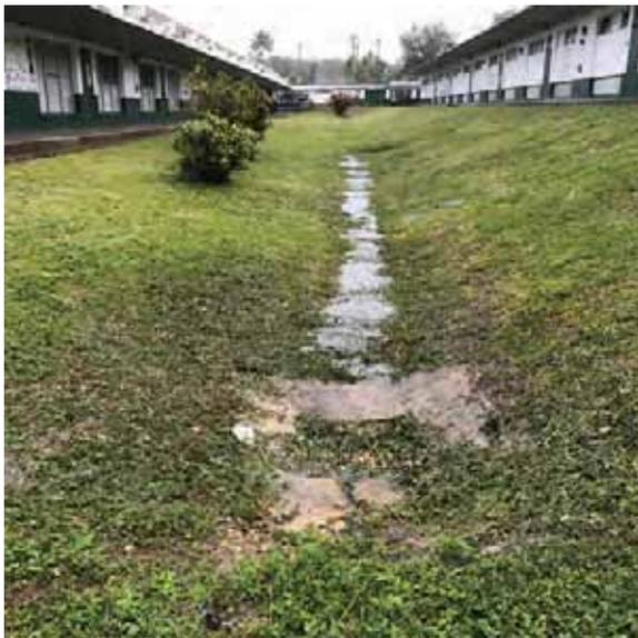
Figure 1: Grass Swale (swales may also be concrete construction)
