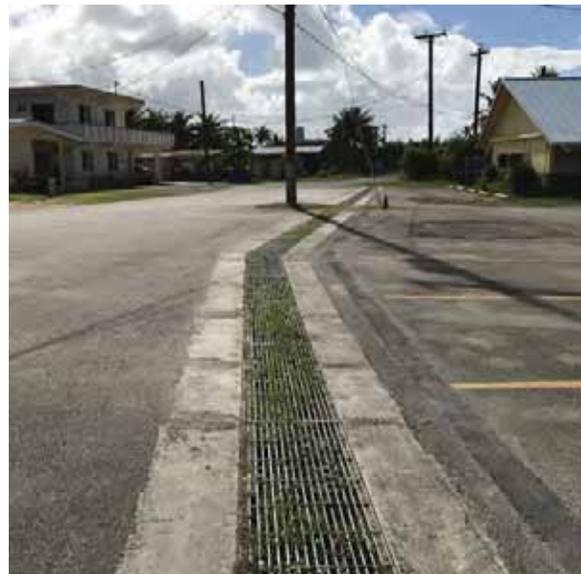
Figure 2: Trench Drain
