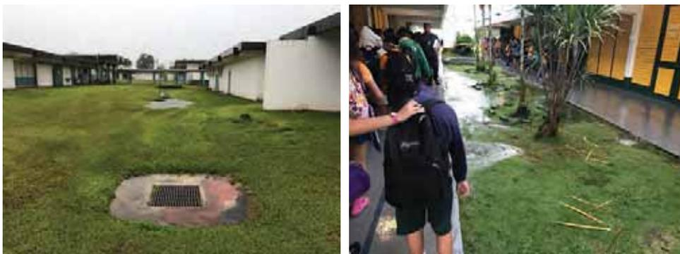
Figure 10: These grass swales do not convey water to the drain inlet or away from the sidewalks and need to be re-constructed.
