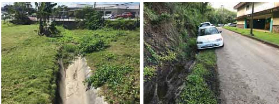
Figure 8: Mud, grass and weeds in concrete and grass swales block the flow of stormwater, causing poor drainage.
